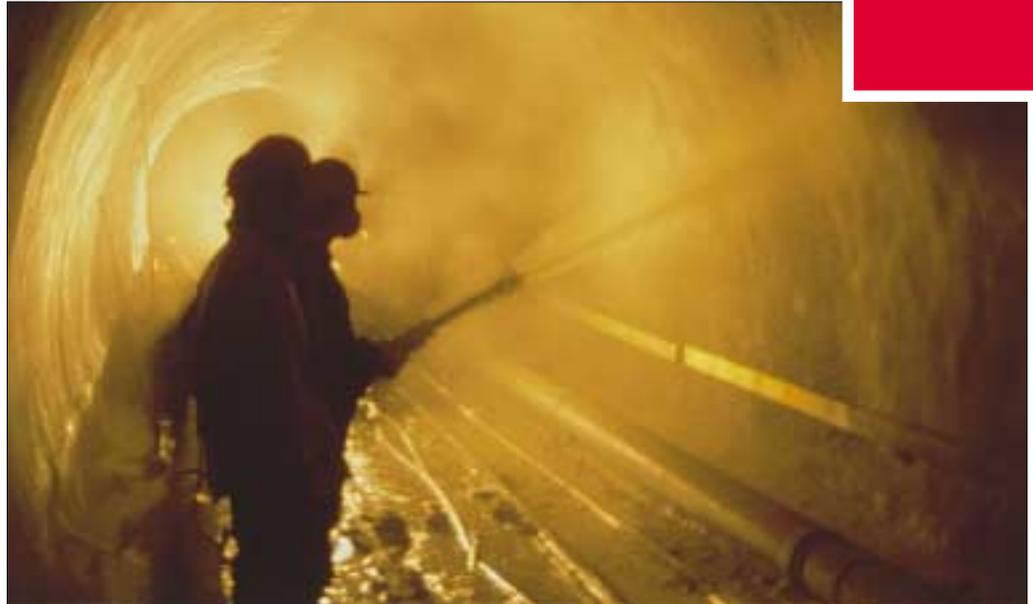
*Dry process shotcrete for tunnel support in soft rock conditions.*
