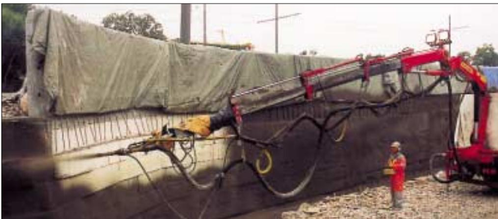
*Wet process shotcrete robot in operation.*
