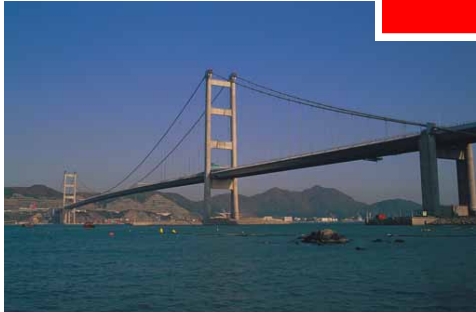
Figure 1. The Tsing Ma bridge in Hong Kong is built in triple blend concrete
